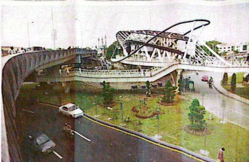
TRAFFIC piles on the newly inaugurated Marka-I-Haq Square in Rawalpindi on Tuesday. — Photo by Muhammad Aam
