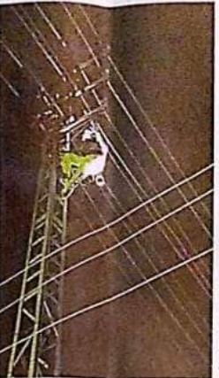
A LABOURER works on a transmission line in Larkana — Dawn
