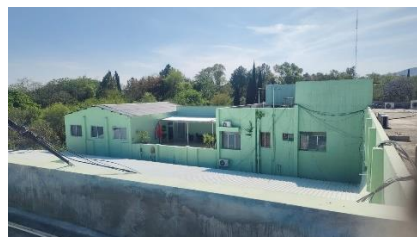
Cable Routing Towards Main Building – Ground Floor
