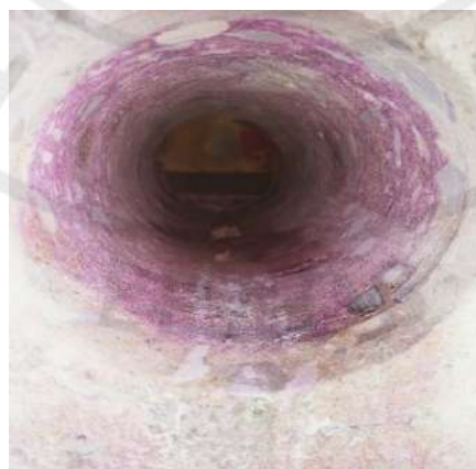
Figure 1: Carbonation Test of The Core
